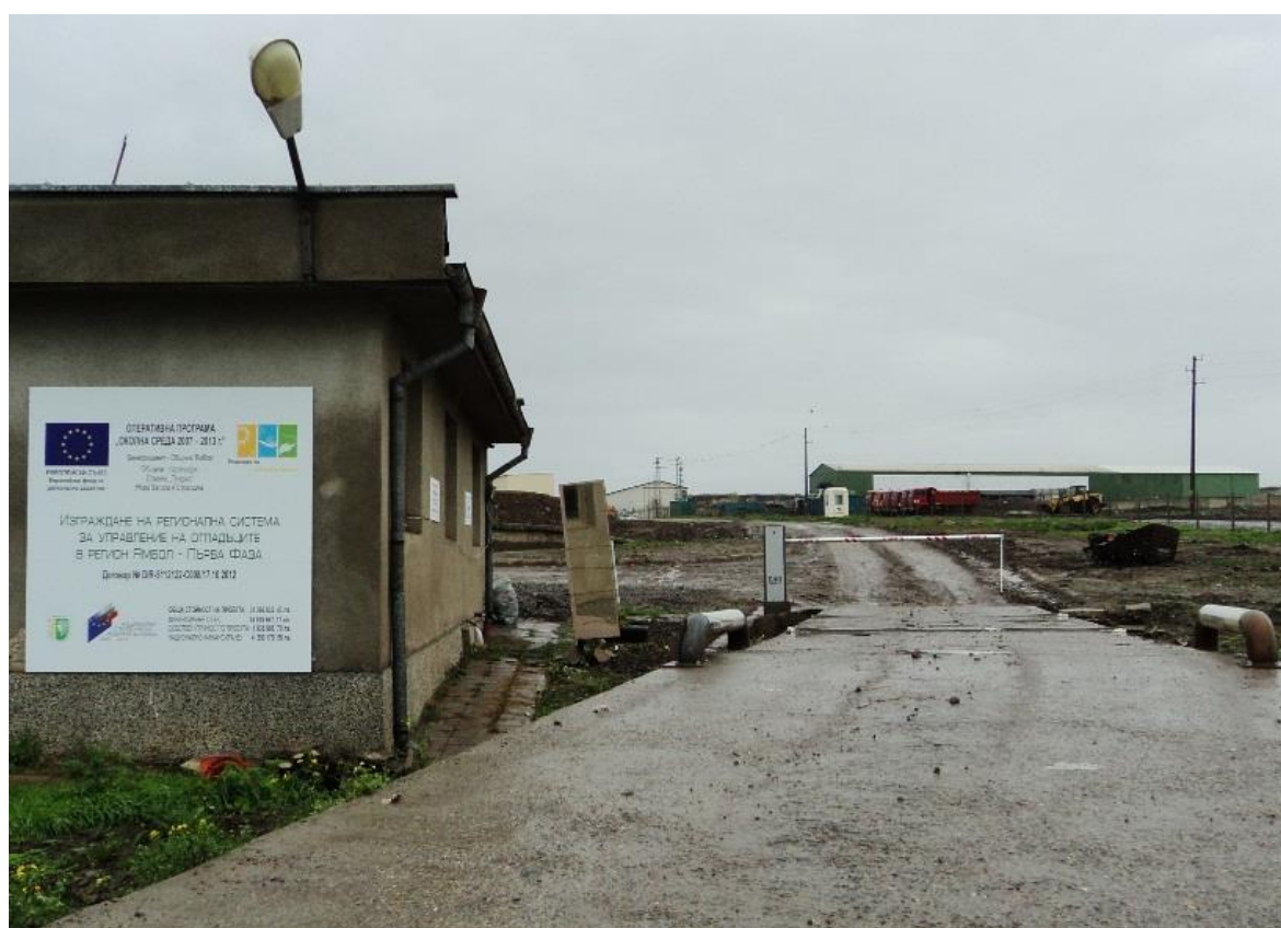
Figure 2 - Entrance to the Yambol landfill in Bulgaria, with Materials Recovery Facility visible in the background
