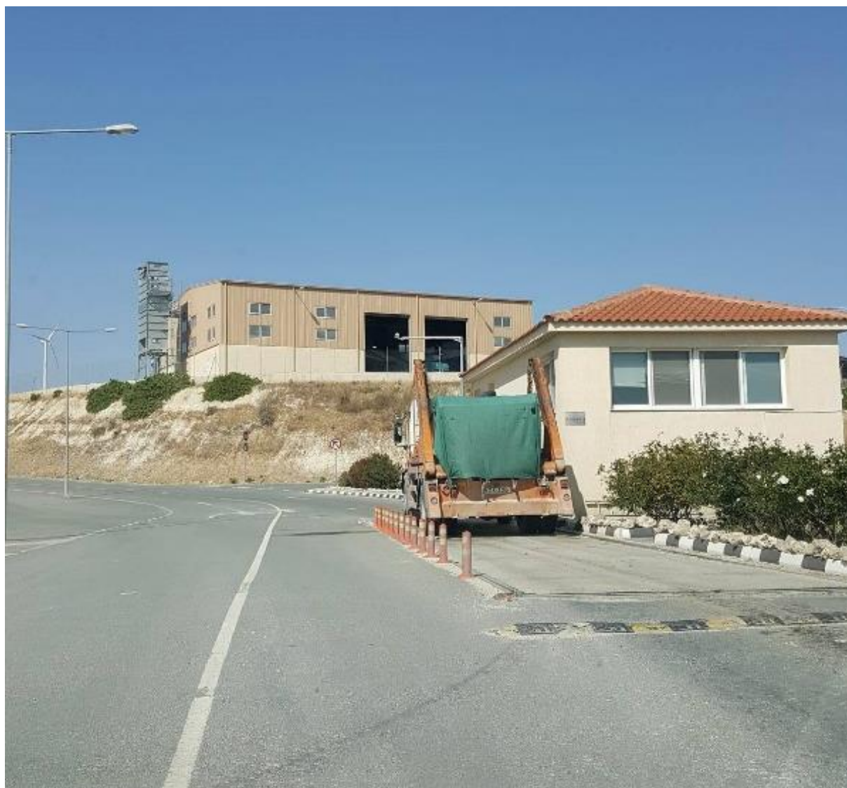
Figure 4 - Weighbridge at the Integrated installations for the management of municipal solid waste, regions of Larnaca – Famagustain, in Cyprus
