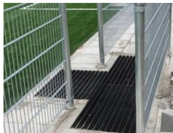
Figure 10. Example of an entrance with a cattle grid to capture rubber granulate.
