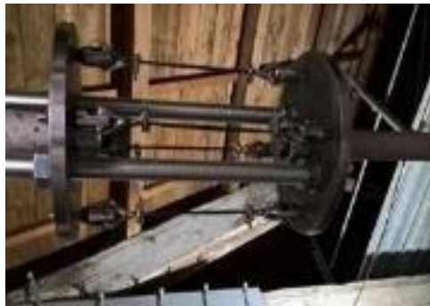
Structural reinforcing & seismic protection
